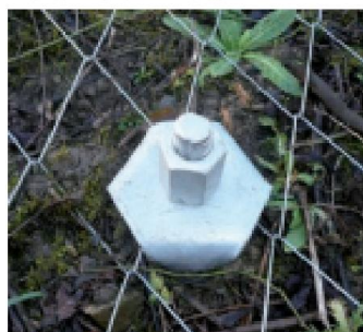
Hexagonal claw plate, for load transfer to mesh
