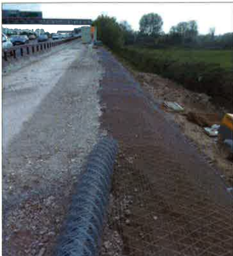
Anchor trench at the crest of the slope
