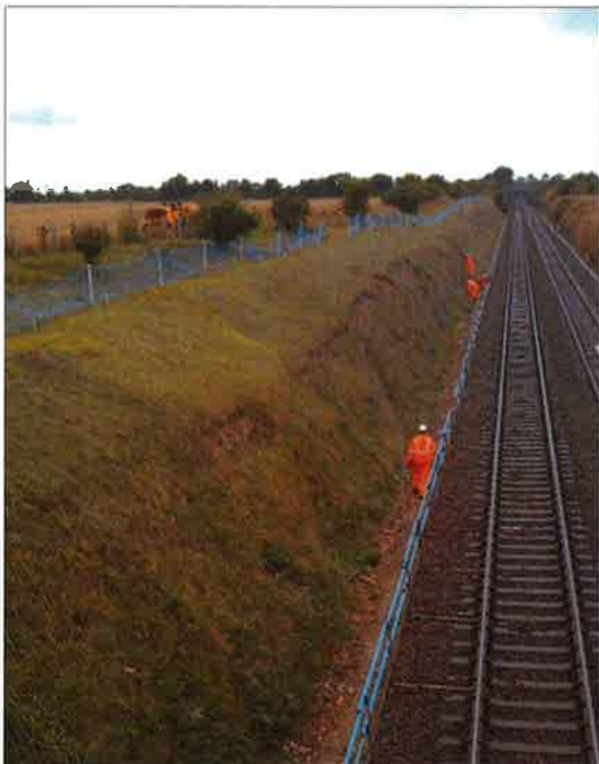
Railway cutting, face stabilisation with DELTAX
