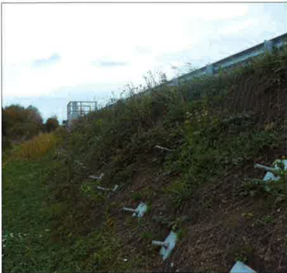
DELTAX mesh and soil nails with re-established growth
