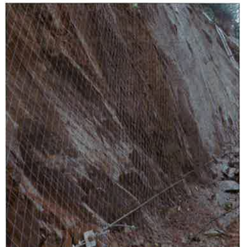
DELTAX drape mesh with GEWI rock bolts
