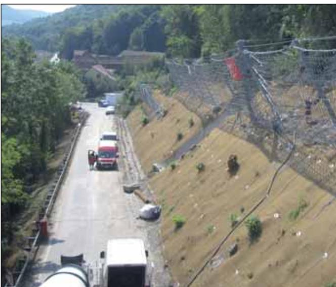
Greenax slope protection mesh, laid below catch fence
