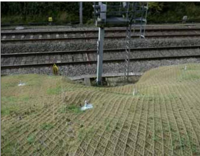
T3 mesh clips used to join edge seams on Greenax
