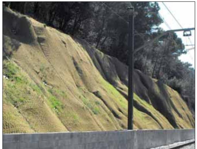
Greenax mesh contoured on slope face, with profiling bolts
