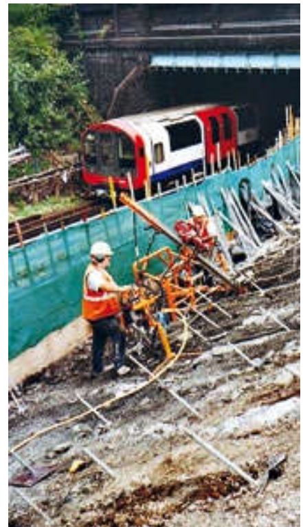
Restricted access soil nailing
