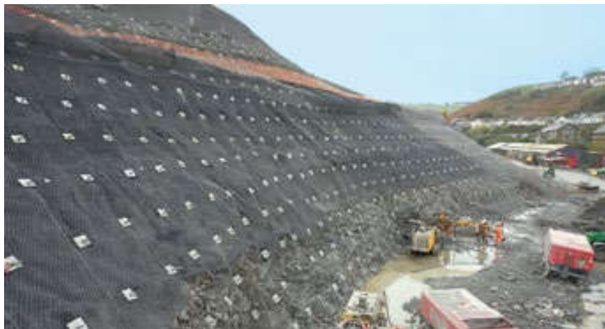
DYWI® Drill Hollow Bar soil nails, top bar galvanized, for slope stabilization
